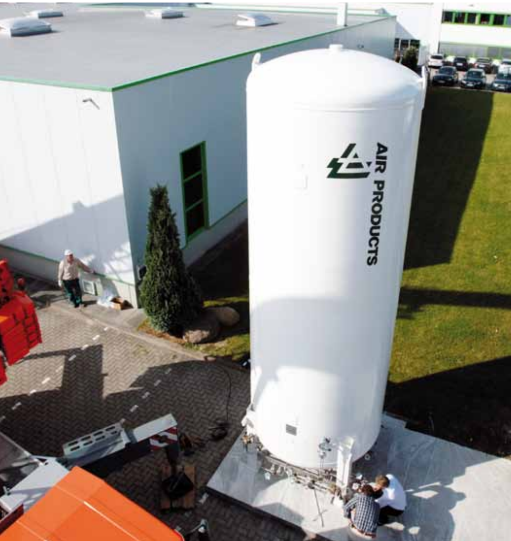
es are being installed
