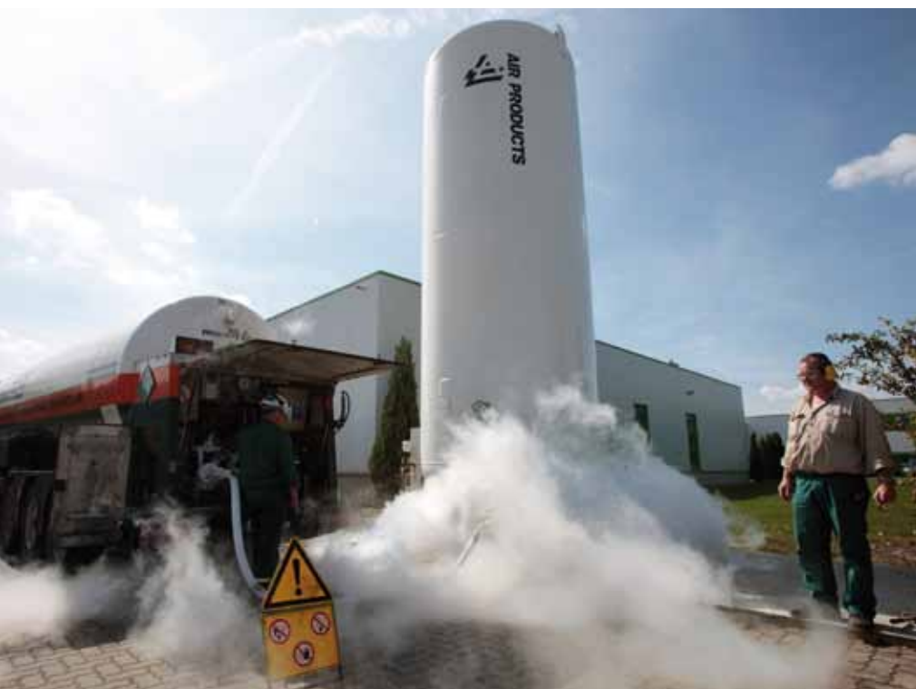
At the end of the day, the tank is filled with oxygen for the very first time
